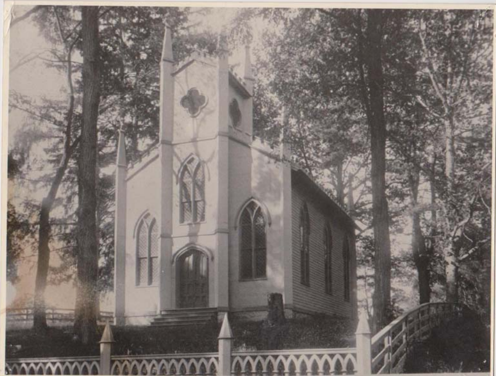
ELLESDIE CHAPEL AT THE ENTRANCE TO BOWDOIN PARK.
